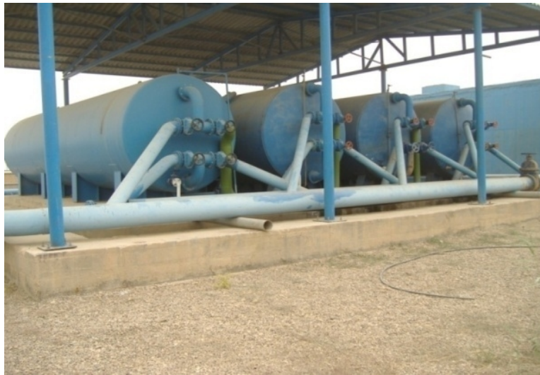
Fig. 1: Under pressure sand filters in the refinery
